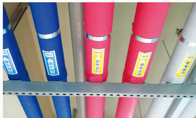
Insulation constructed with magic tape for PIPE
