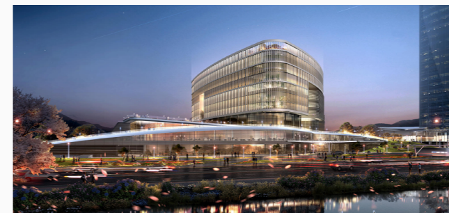
Health Insurance Review and Assessment Service Office Building 2 In Wonju, Korea
