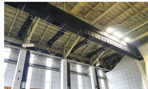
Air conditioning & ventilation facility DUCT construction
