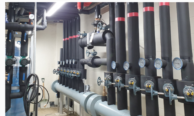
Mechanical facility PIPE construction
