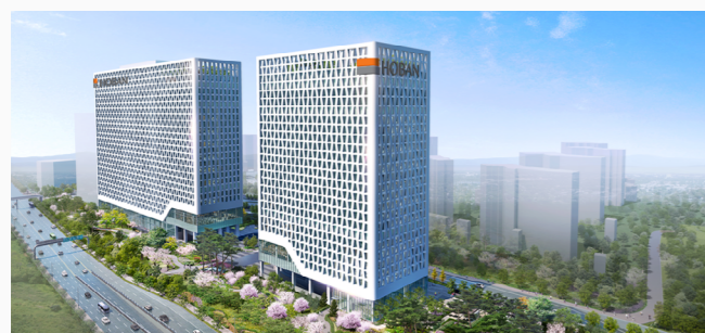
Hoban Construction Company New Office Building in Seoul, Korea
